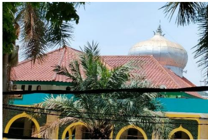
Figure 8. Mosque Roof (current)
